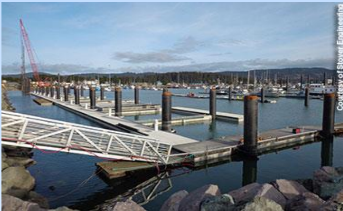
March 2014: Rebuild in "tsunami resistant" Crescent City Harbor
